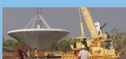
Lifting the dish at Katherine on December 3 2009.
